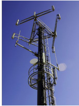
Figure 1.1: Base station antenna(Global Distributed Antenna Systems Market, Global Distributed Antenna Systems Industry: Ken Research).
